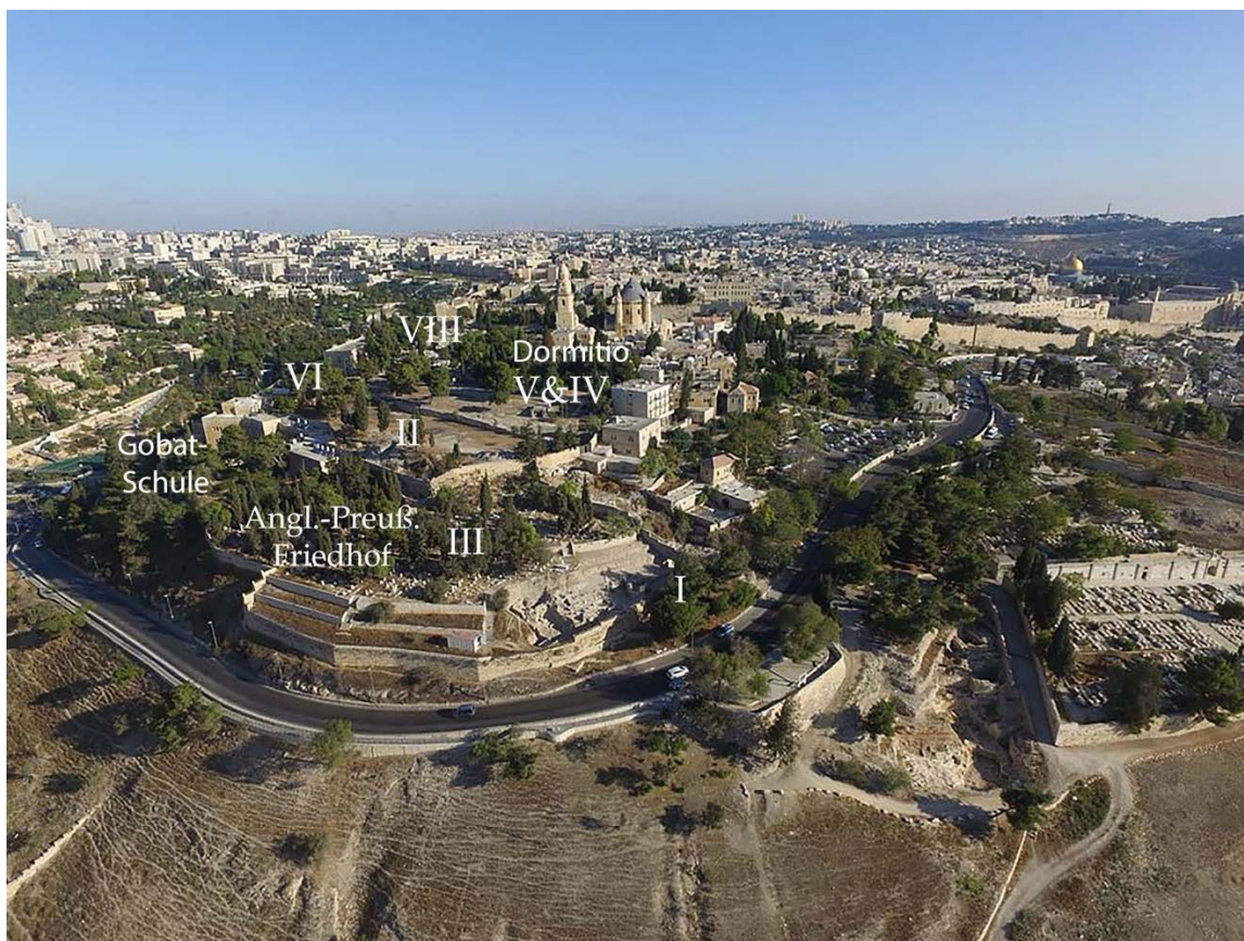
Fig. 1: Mount Zion (southwest hill) of Jerusalem; view from the south with the excavation areas of the GPIA and the Dormitio Abbey in the foreground and the Old City in the background © Yehiel Zelinger, IAA
